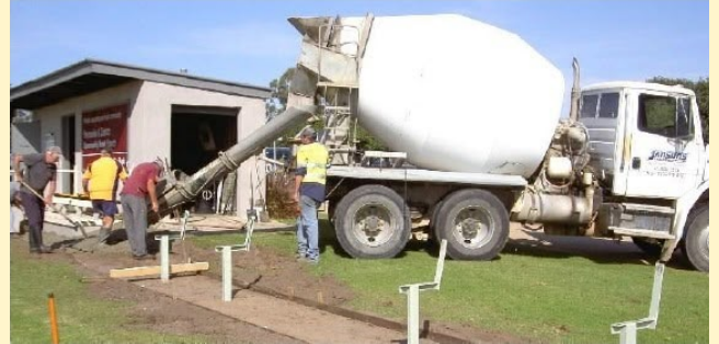
It was all hands on deck when the truck arrived! Steve Beggs, Alan Werner, Mick Blackwood, Graeme White and Peter North were very active getting the job done.
